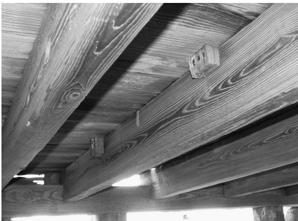
FIGURE 40. View of connection of wall studs and floor joist on east side of Room 101. (NPS-SERO-CR, 2003)
