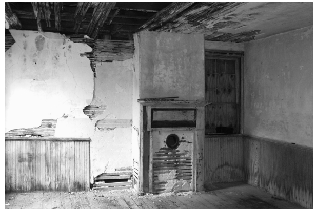
FIGURE 18. View of chimney in Room 103, absence of wainscot indicating extent of original chimney. (NPS-SERO-CR, 2003)
