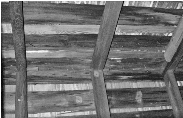
FIGURE 45. View of typical rafter connections at ridge. (NPS-SERO-CR, 2002)
