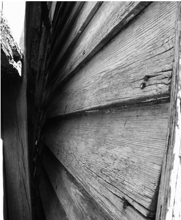
FIGURE 52. View of original beaded siding remaining on north west side of main block at kitchen addition. All of this siding was replaced in 2003. (NPS-SERO-CR, 2002)
