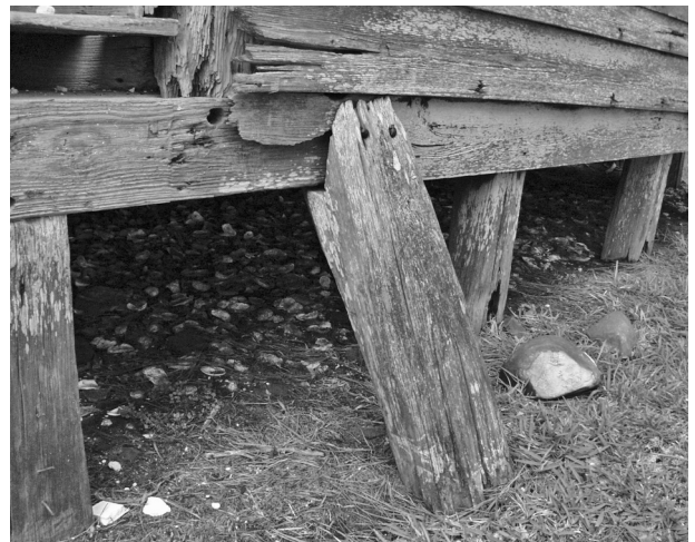
FIGURE 35. View of a typical "bird's-mouth" hurricane brace on north side of house. (NPS-SERO-CR, 2002)
