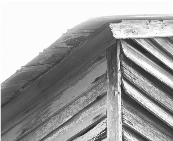
FIGURE 53. View of north corner of house, showing typical treatment of eaves and corners. Light areas appear to be paint but may actually be due to the presence of lichen or other natural discoloration. (NPS-SERO-CR, 2002)
