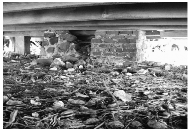
FIGURE 36. View of chimney foundation, with brick at right marking existing chimney base and stone at left marking larger extent of original chimney. (NPS-SERO-CR, 2002)
