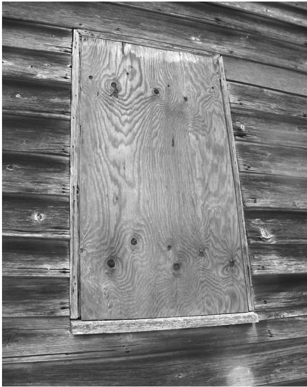
FIGURE 49. View of W-1 with original exterior sill and casing intact. (NPS-SERO-CR, 2002)
