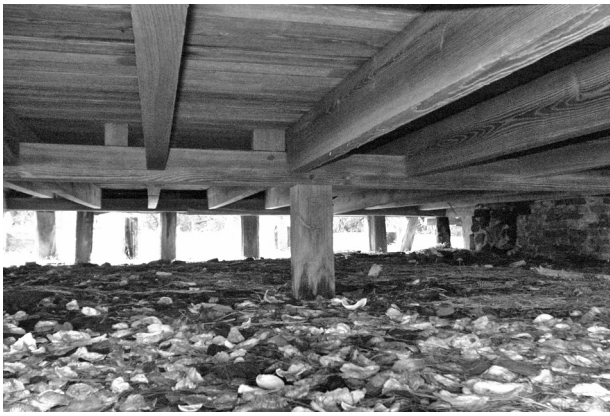
FIGURE 37. View southwest under main block of house, showing shells used to stabilize the ground under the house. (NPS-SERO-CR, 2002)
