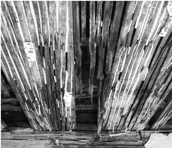
FIGURE 56. View of ceiling in Room 101, showing typical split-board plaster lath. (NPS-SERO-CR, 2002)
