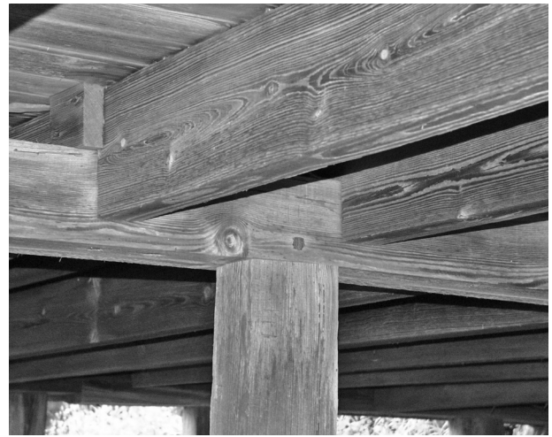
FIGURE 34. View of typical joist and pier connections at center beam. (NPS-SERO-CR, 2002)
