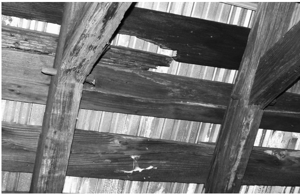
FIGURE 44. View of typical connection of collar beams and rafters. (NPS-SERO-CR, 2002)
