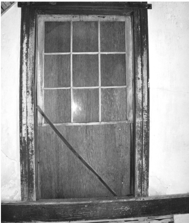
FIGURE 50. View of W-2 with sash and trim typical of first floor windows. (NPS-SERO-CR, 2002)
