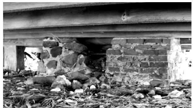
FIGURE 20. View of chimney base, with original stone chimney base at left, existing brick chimney at right. (NPS-SERO-CR, 2003)
