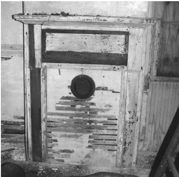
FIGURE 63. View of fireplace and mantel in Room 103, probably installed along with construction of the kitchen wing in the late nineteenth or early twentieth century. (NPS-SERO-CR, 2002)
