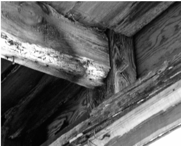
FIGURE 39. View of typical connection of second floor joists and studs. (NPS-SERO-CR, 2002)
